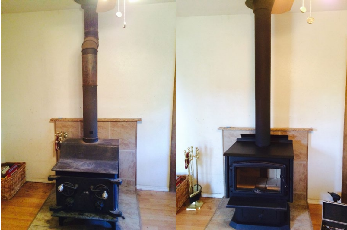
Figure 3. Example of Before (left) and After (right) Pictures Collected as Part of the Documentation for Change-out 2016-011
